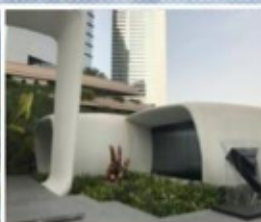
The 3D Printed Office of the Future, Dubai, UAE
